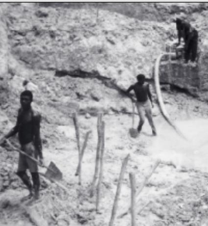
A small pump drains an alluvial diamond pit. Photo: Des Garvey.
