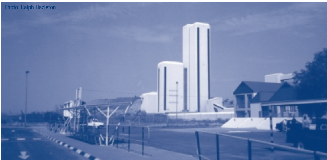
“The Aquarium”, Treatment Plant at Jwaneng Mine, Botswana
